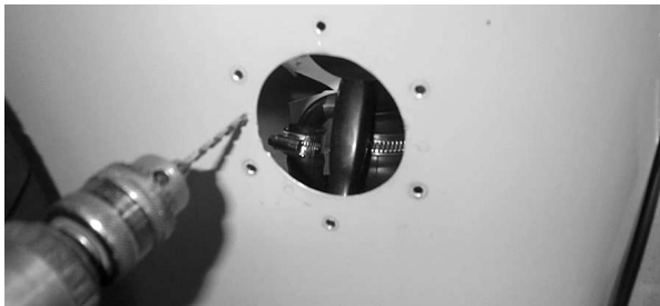
Fig 17 Carefully drill new holes
