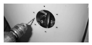
Fig 17 Carefully drill new holes
