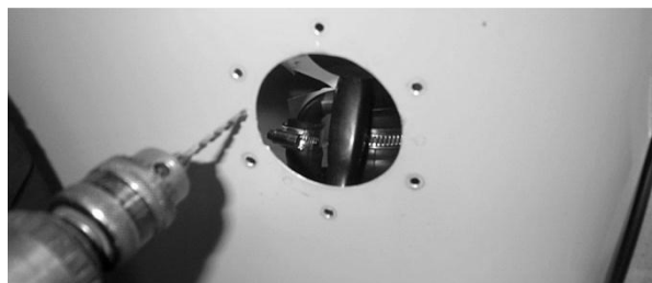
Figure 186: Carefully drill new holes
