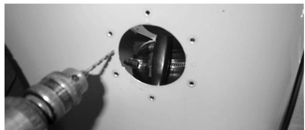
Figure 186: Carefully drill new holes
