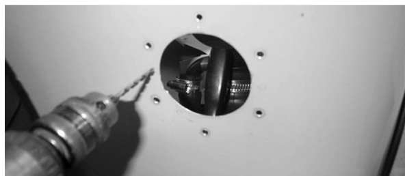
Figure 191: Carefully drill new holes
