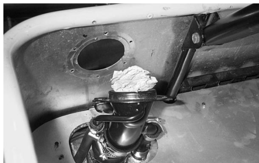
Figure 190: Old filler boss removed
