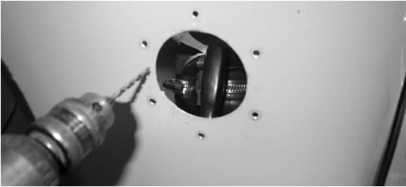
Fig 17 Carefully drill new holes
