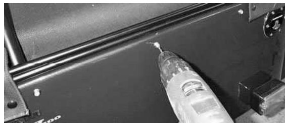
Fig 22 Drilling central popper on SV
